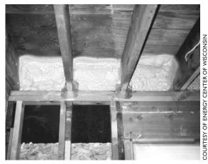
(above left) Wood rot—the result of moisture getting into the attic. (above right) Spray-in insulation can prevent condensation on inside walls. (left) Ice dams are caused by poor insulation and air leaks between the ceiling and attic.
