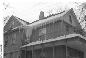
Even dry indoor air can cause problems by causing ice dams. Most ice dams form when heated air from the house escapes into the attic and warms the underside of the roof, causing snow to melt and then refreeze when the water hits the cold overhang. Ice dams can force water back into the attic, where it can soak insulation and damage ceilings. Sealing leaks between the house and the attic is important for preventing both types of problems.
